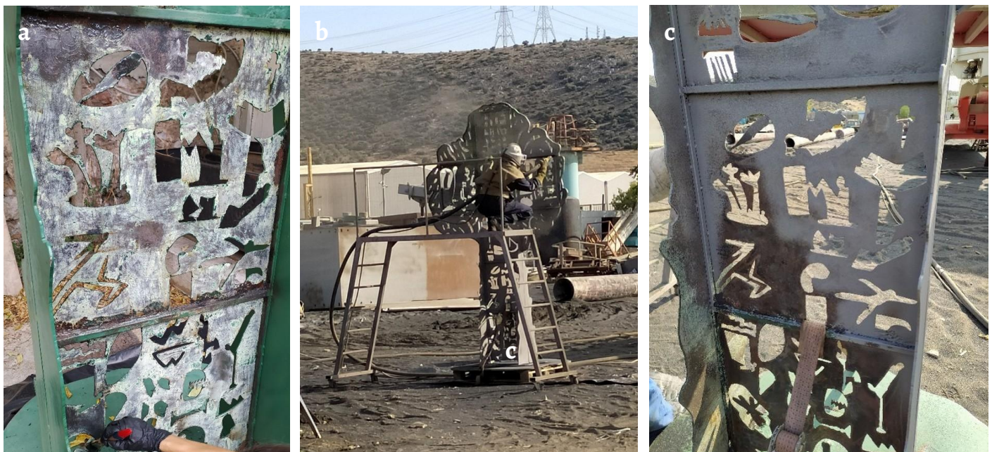
Figure 6. Mechanical cleaning of paint layers: a) cleaning result of paint layers with commercial paint remover and a hot air gun; b) cleaning with an industrial air blast system; c) view of a cleaned area with the sandblasting system, revealing the blackening of the surface due to the process of metal cutting for creating the symbols. The details of the cutting of the symbols are better observed.
