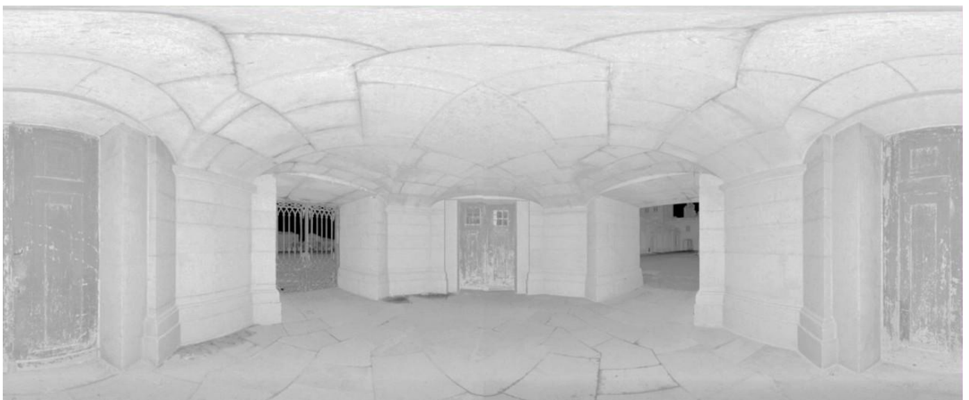
Figure 2. Panoramic view of the vault, obtained from laser scanning. It shows two openings (to the main façade of the palace and to the yard) and connections to interior of the palace.
