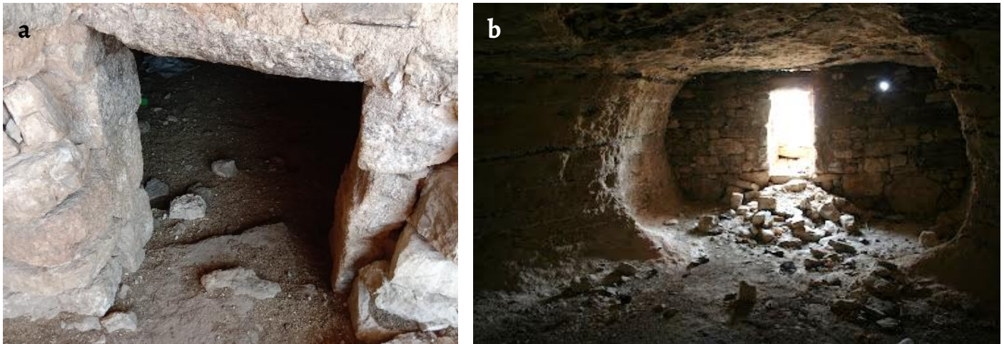
Figure 8. Abandoned and misused hermit caves that surround Machaerus Fortress, 2022: a) an interior view revealing stone collapse and physical deterioration; b) a cave interior demonstrating accumulated debris, lack of conservation, and ongoing neglect.
