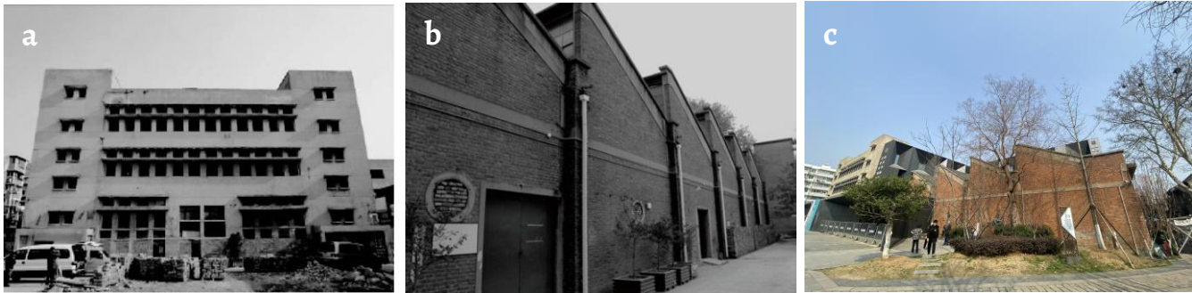
Figure 9. Nanjing Yarn-dyed Fabric Mill: a) from the perspective of Jianzi Alley; b) view of the industrial buildings with the zigzag roof; c) Jinling Art Museum.
