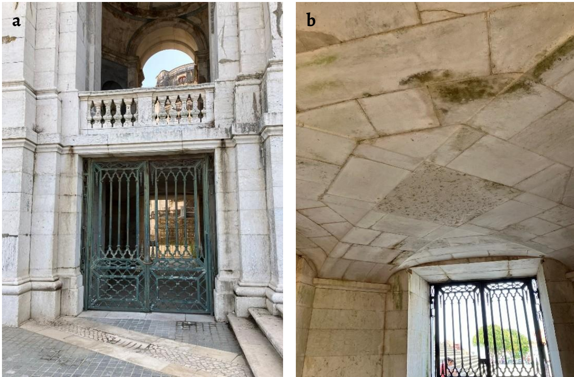
Figure 1. Vault: a) location of the vault in front facade; b) bottom view under the vault.
