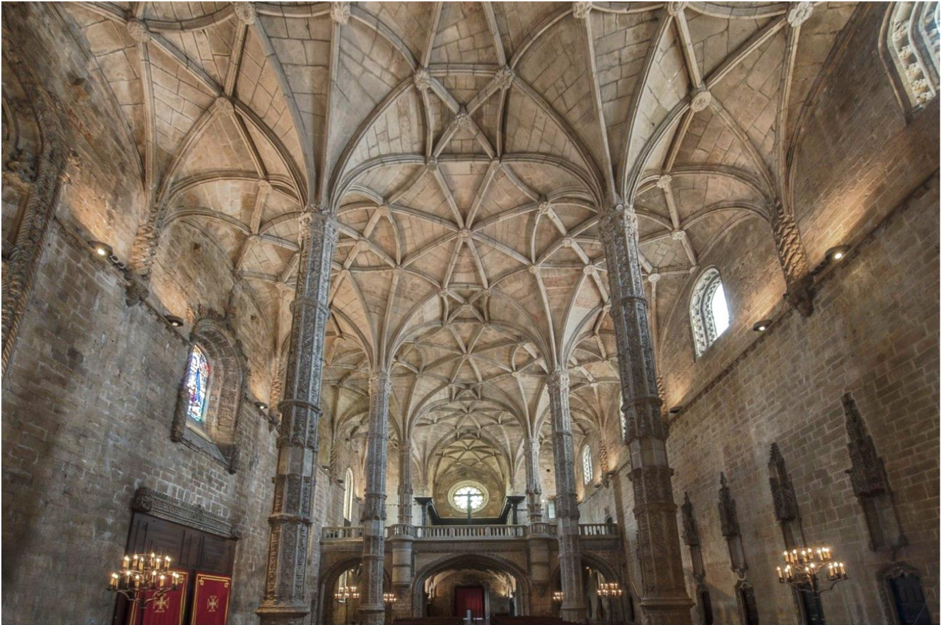
Figure 6. Church, nave vaults, 2013 (photo: A. Serralheiro).
