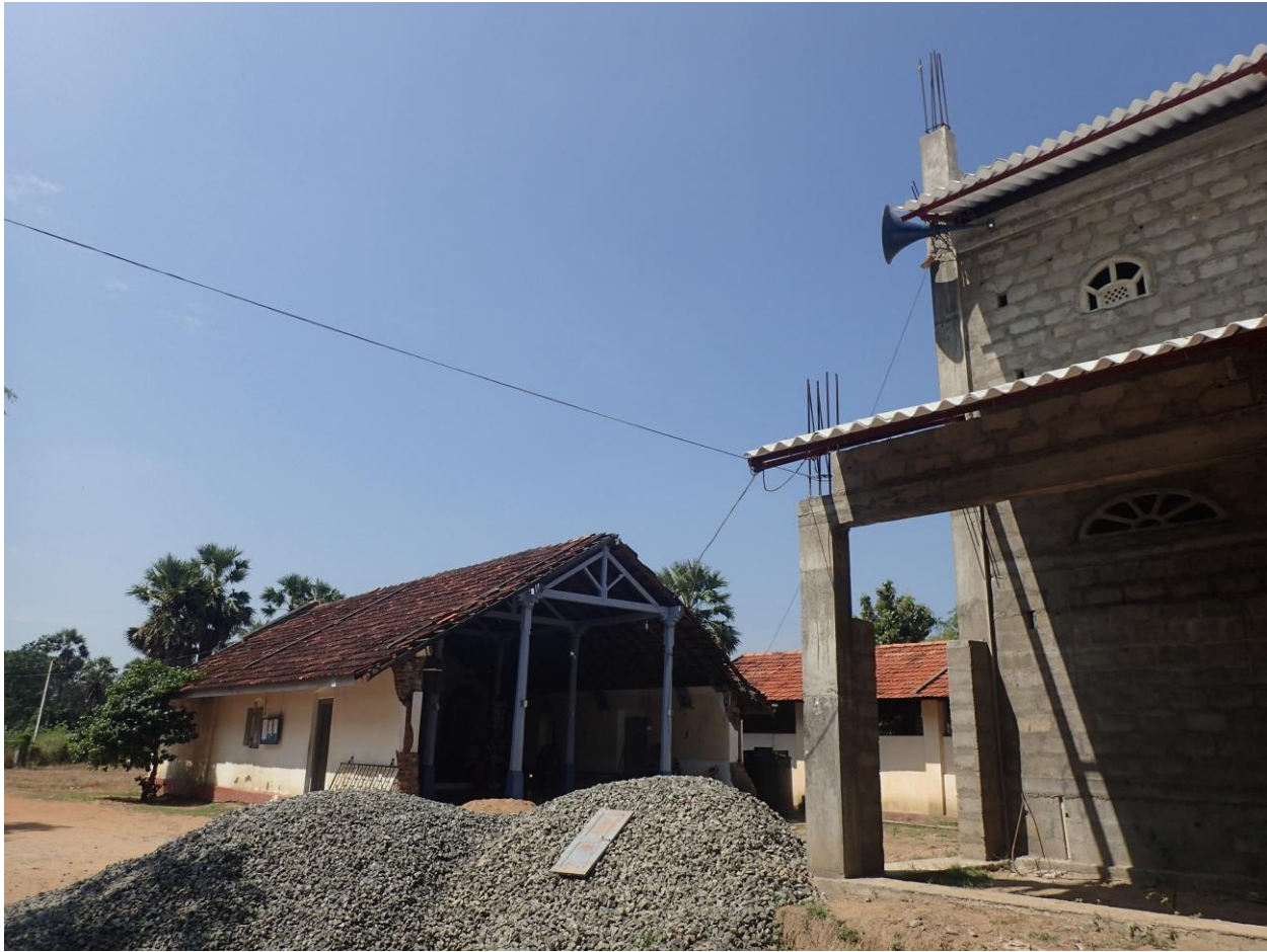
Figure 3. Holy Rosary Church in Palayadipudikulam, Mannar, in 2018 during its demolition, while the new church was being constructed in front of it (photo: Joaquim Rodrigues dos Santos).
