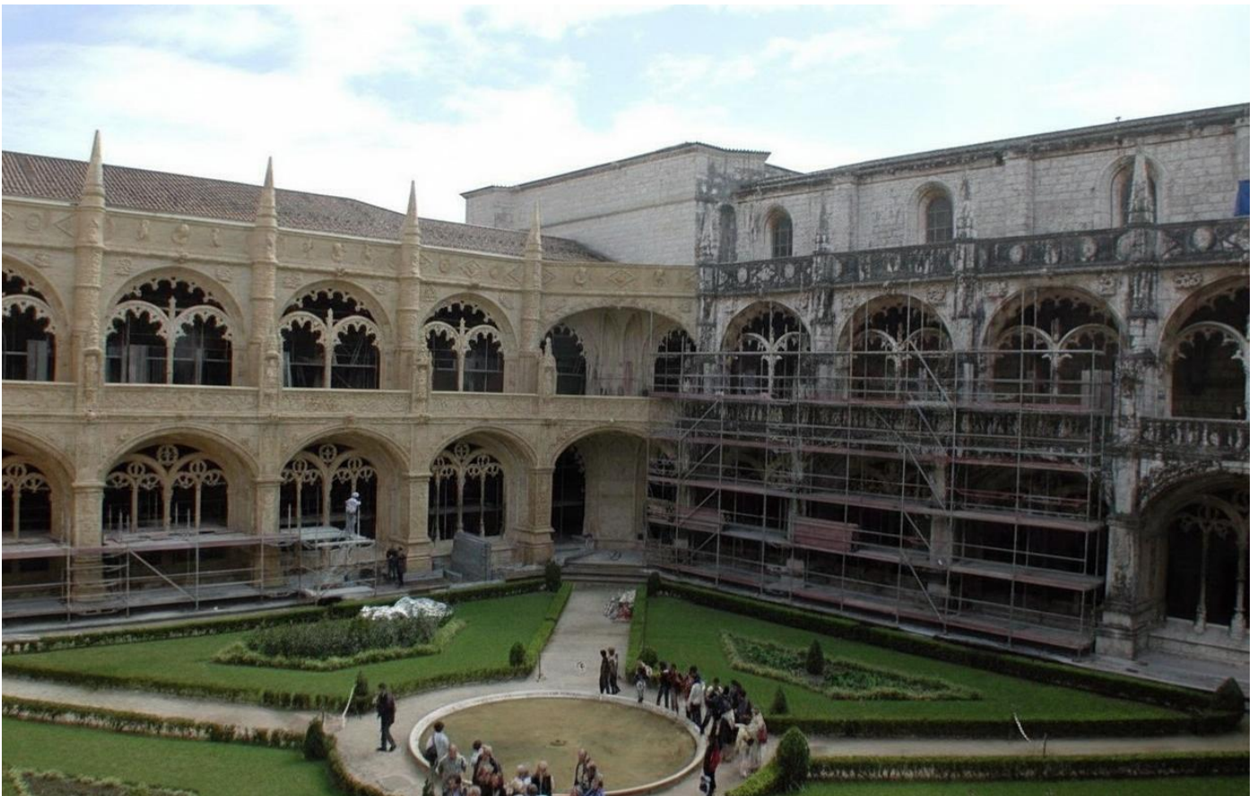
Figure 5. Ongoing works in the cloister, with visitors contemplating the intervention, c. 2000 (photo: D. Caldeira).
