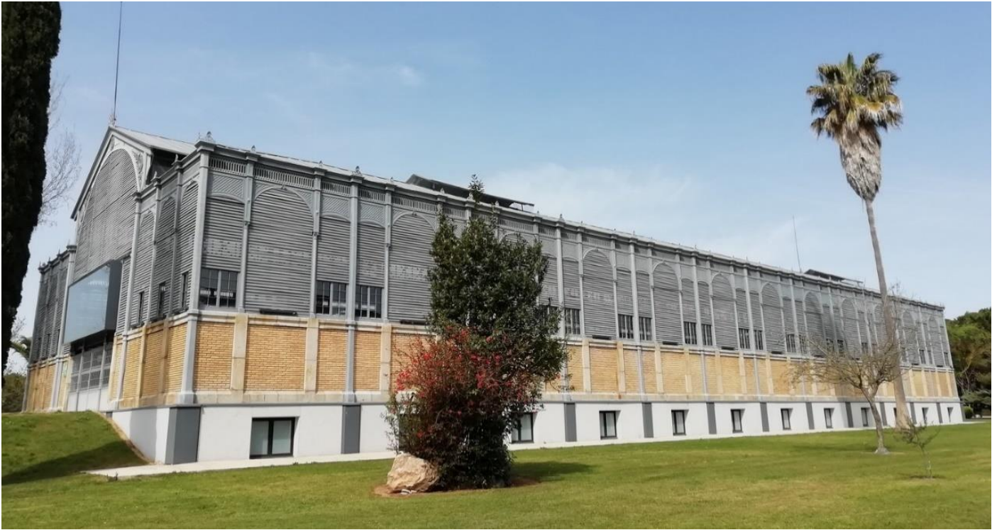
Figure 6. External view of the old Badajoz food market, Universidad de Extremadura, Badajoz (photography: Sheila Palomares Alarcón, 2021).
