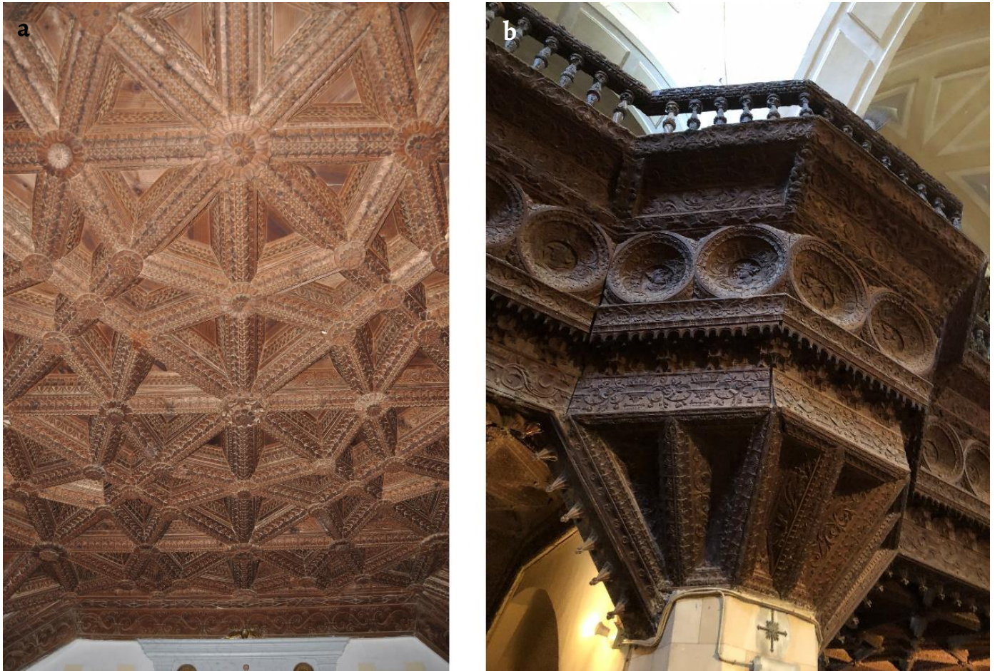
Figure 5. Gallery of the choir: a) ceiling; b) front.
