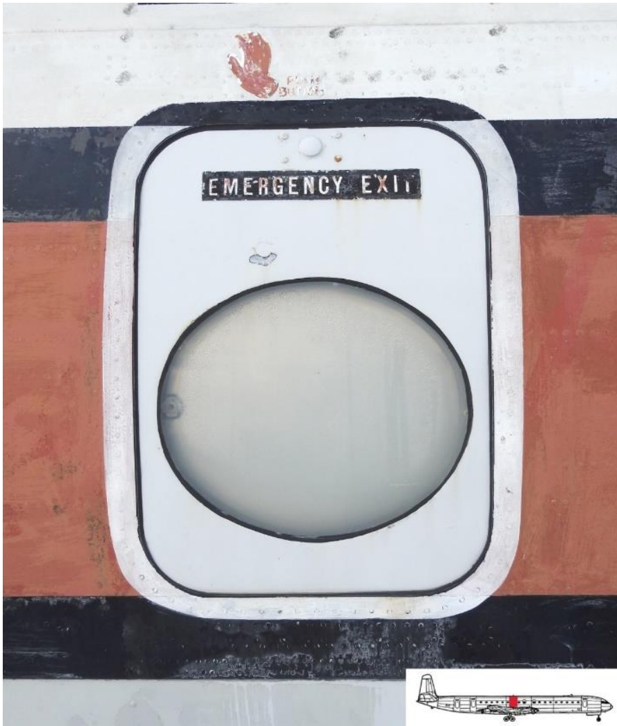
Figure 9. Recurrent corrosion on emergency exit window.
