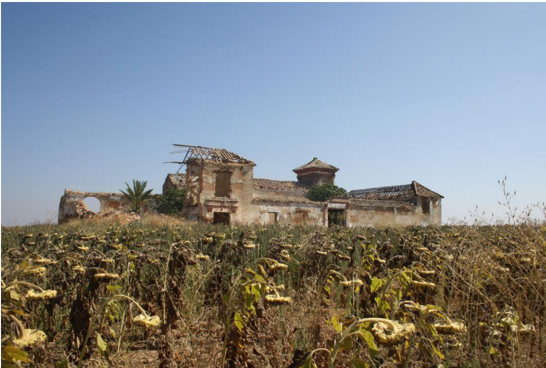
Figure 4. Charcón mill in Écija. It still contains the robust counterweight tower characteristic of beam and weight presses.
