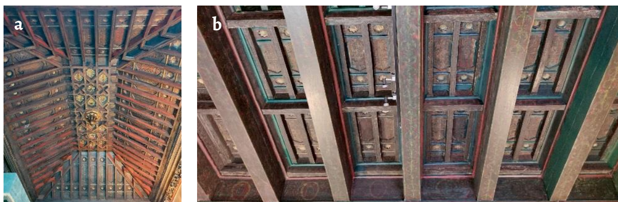
Figure 14. Ceilings: a) chapel's original coffered ceiling; b) coffered ceiling transferred to the antechapel. Authors' photographs (2021).
