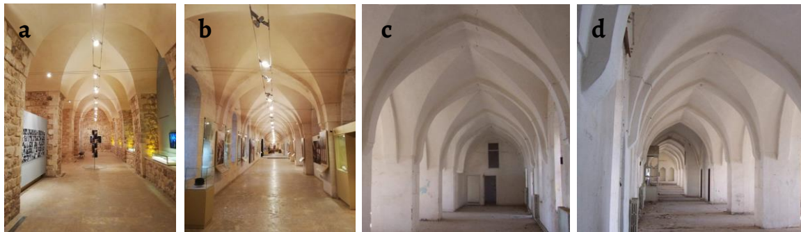
Figure 8. a, b ) Interior view of the building used as a museum (2020), photographs by İzzettin Kutlu and c, d ) interior view of the building used as Tax Office (2000s), photographs by Murat Çağlayan.
