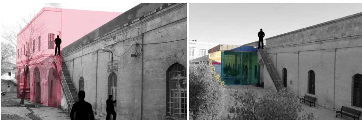
Figure 7. a) Representation of the first floor and portico of the building in its original state, b) The glass-steel construction entrance hall with glass-steel construction referring to the portico of the northern entrance door (2020), photographs produced İzzettin Kutlu.
