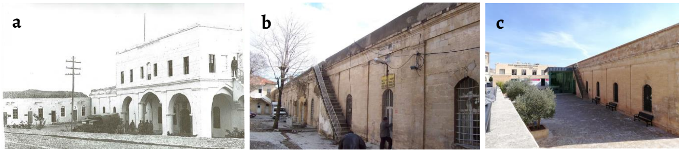
Figure 10. Chronological views of the North facade of the building that has undergone the most change a) 1900s, b) 2004, and c) 2019.
