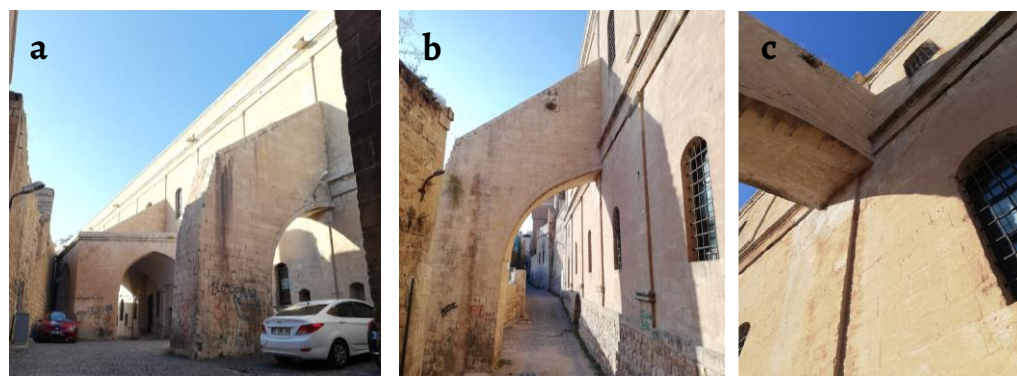
Figure 4. Today's views of the 4 buttresses added, photographs 2020 by İzzettin Kutlu.
