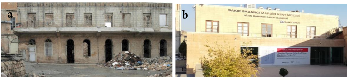
Figure 6. a) Demolished old storage and b) new contemporary addition building views, photographs by Şanlıurfa Regional Board of Conservation of Cultural Heritage.
