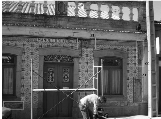
Fig. 1 Mortar sampling, showing different sampling areas
