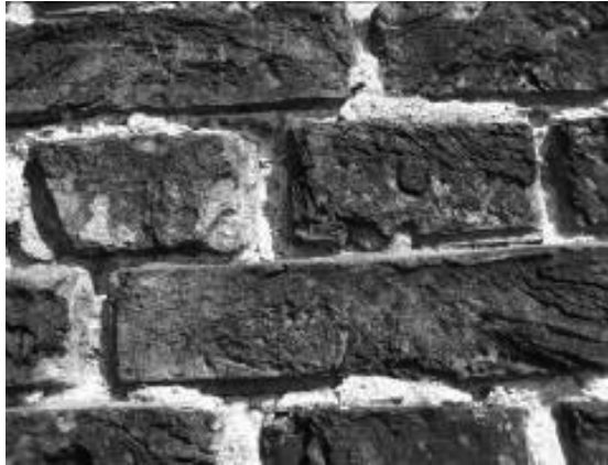
Fig. 3 Above, outside weathered side face of brick and inside (not weathered) original bed face of brick; below, outside weathered side of a wall.
