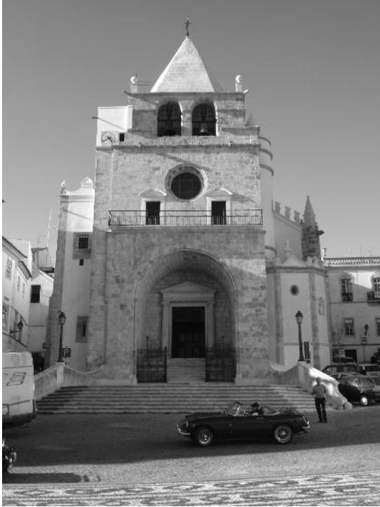
Fig. 27 The main façade after the conservation and restoration works of the historical mortars.
