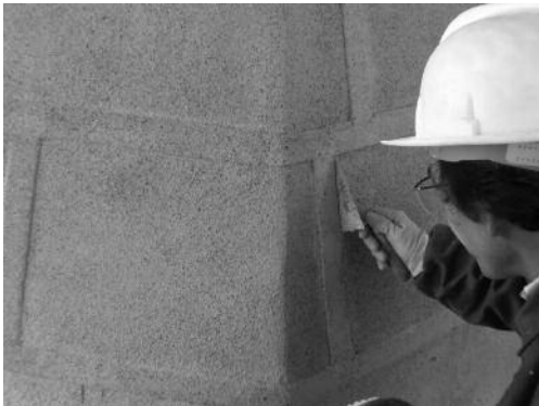
Fig. 23 Detail of the application of the final decorated layer with raised joints.
