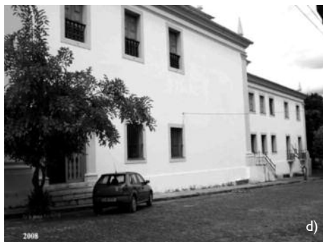
Fig. 12 a) Coating tests; b) After the application in 2006; c) Situation 2007; d) Condition in 2008.
