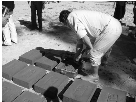
Fig. 4 Oliveirinha, workshop V ATP, the adobe production. Earth stabilized with lime.
