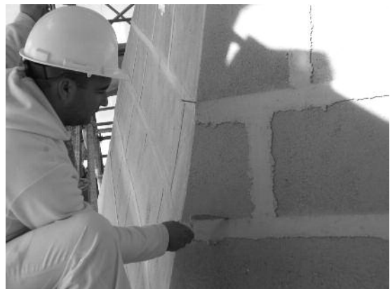
Fig. 21 Removing and cutting, after a first drying, the excess mortar, according to the decorative scheme.
