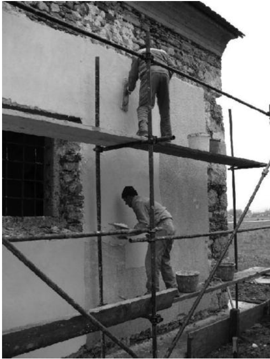
Fig. 11 .Application of finishing layer (two-coat work).
