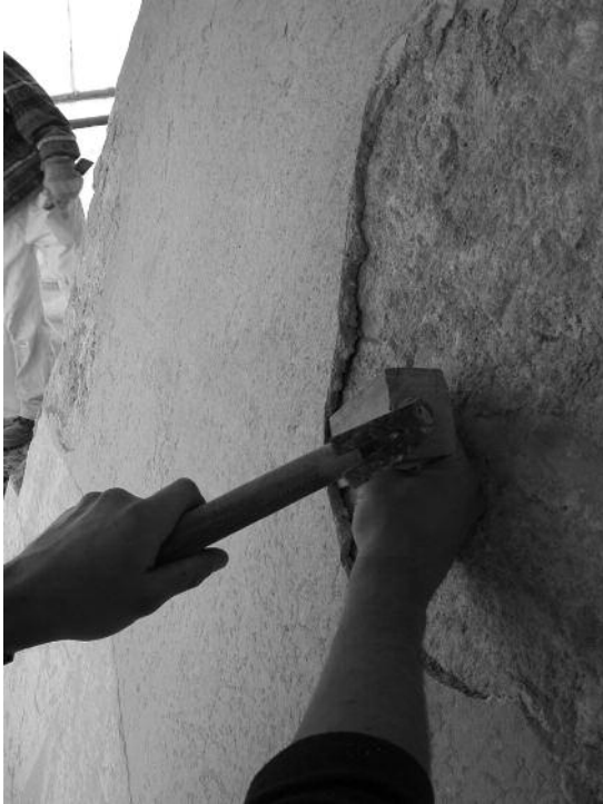
Fig. 5 Removal of the non decorated recovering render.
