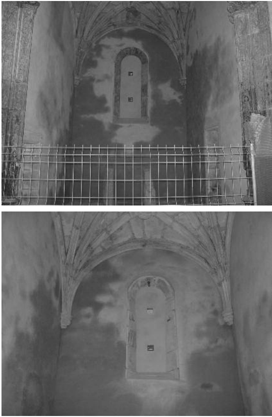
Fig. 4 Drying of a lime-base rendering inside a church in Northern Portugal (September 2004 and January 2005).
