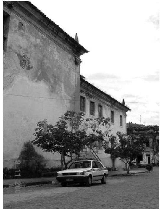
Fig. 11 Situation before the restoration (2001).
