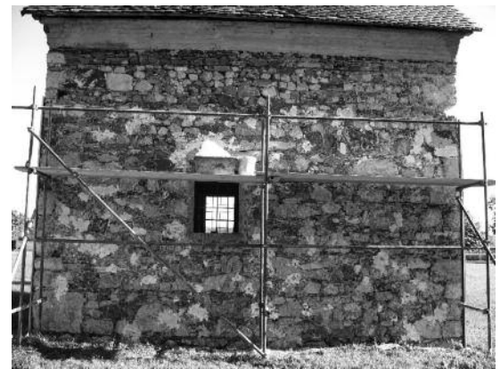
Fig. 2 The test wall after filling of voids.
