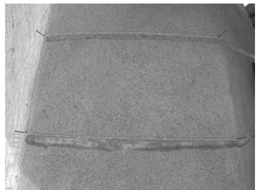
Fig. 15 Reproducing the decorative scheme. The joints were traced using nails and coloured threads.
