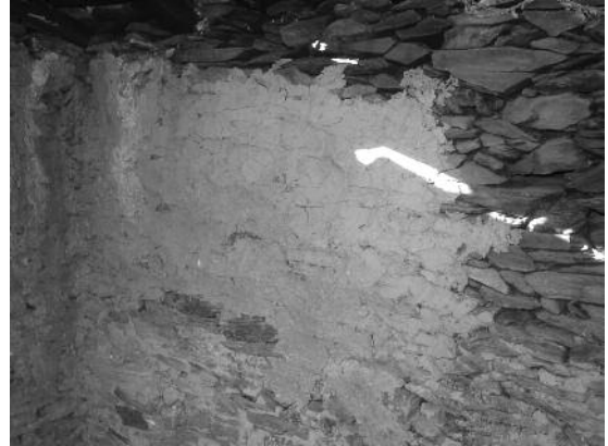
Fig. 2 Mozinhos – Penedono, indoors earth render.
