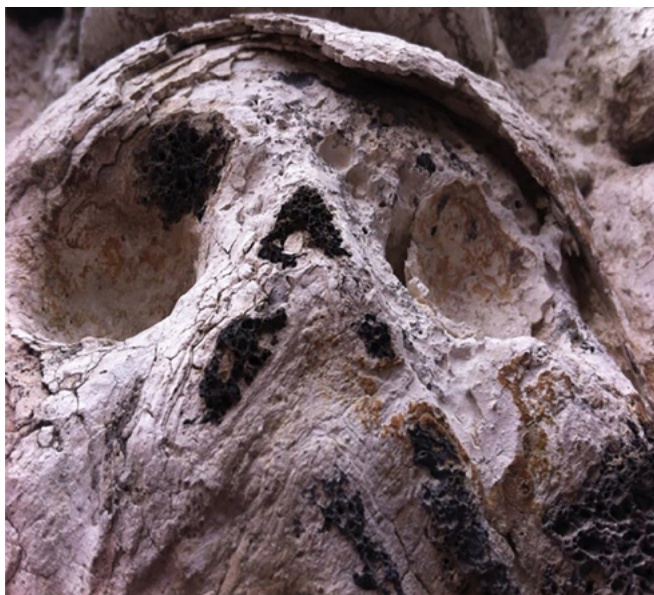
Figure 2. Structure B's stucco pathology example.
