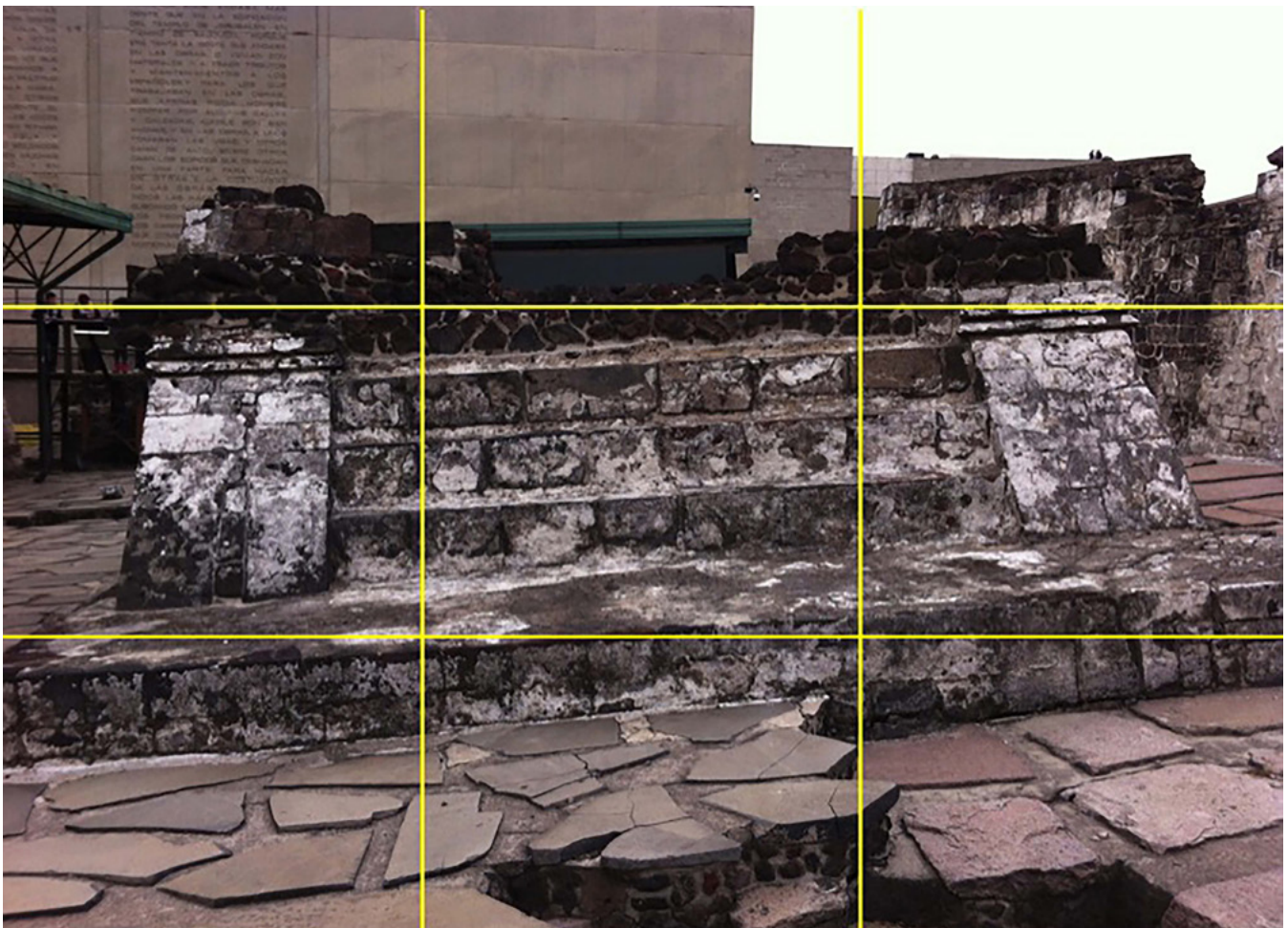
Figure 1. Inclination of the courtyards and Structure B.
