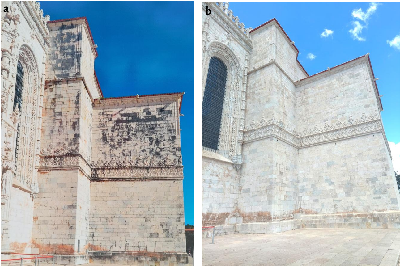
Figure 8. Southern transept chapel façade: a) before and b) after the intervention, 2024.
