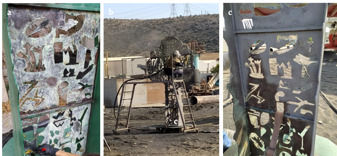
Figure 6. Mechanical cleaning of paint layers: a) cleaning result of paint layers with commercial paint remover and a hot air gun; b) cleaning with an industrial air blast system; c) view of a cleaned area with the sandblasting system, revealing the blackening of the surface due to the process of metal cutting for creating the symbols. The details of the cutting of the symbols are better observed.
