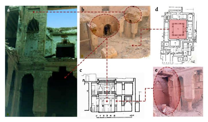
**Figure 10.** 2D restitution, produced from in situ metric and photographic surveys before 3D modelling: *a*) old photos of parts now disappeared; *b-e*) recent photos show parts completely disappeared; *c-d*) sectional and plan survey.
