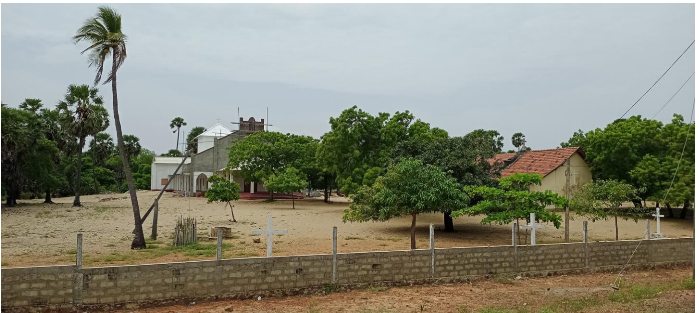
Figure 13. St Bartholomew's Church in Olaithoduvai, Mannar, and the construction of the new church (photo: Sagara Jayasinghe).
