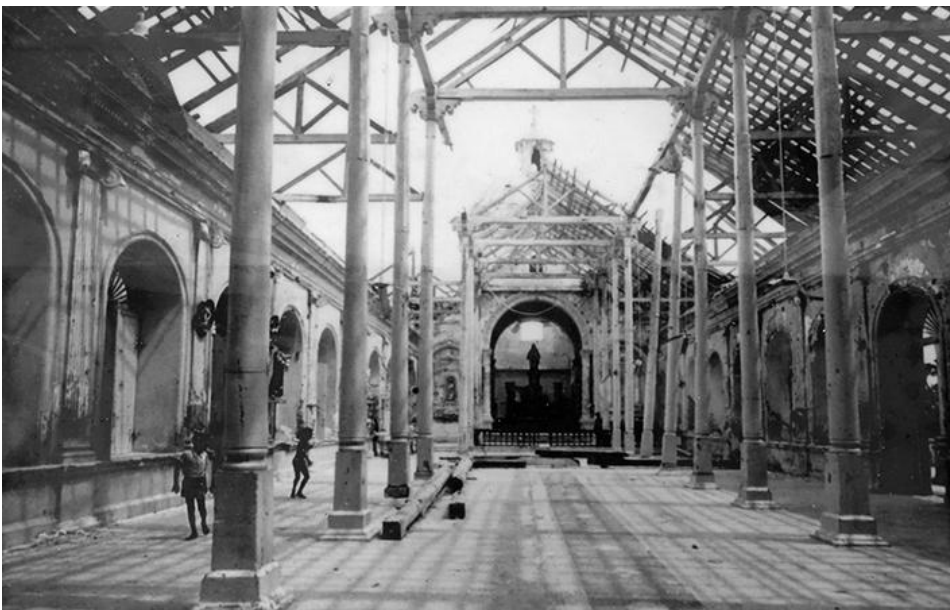
Figure 2. Inside of St James’ Church in Gurunagar, Jaffna, in 1993 after the aerial bombing during the civil war (1983-2009) (source: courtesy of the Parish Priest, St James’ Church in Gurunagar).
