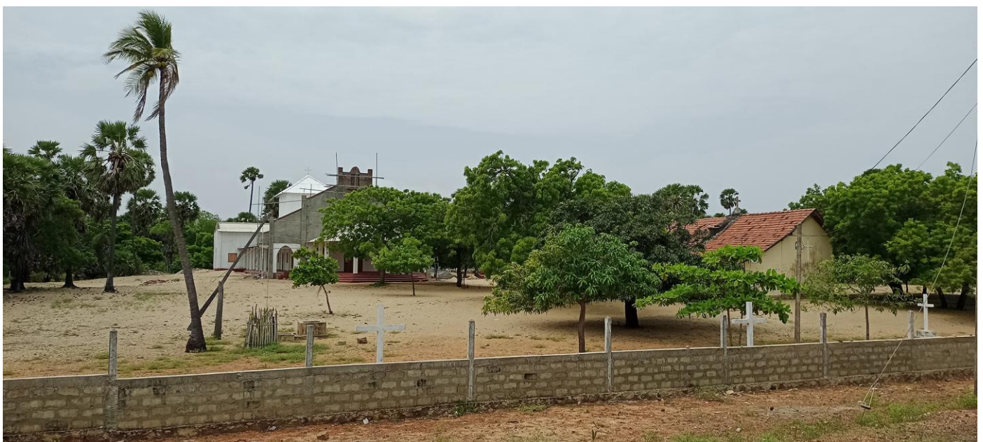
Figure 13. St Bartholomew's Church in Olaithoduvai, Mannar, and the construction of the new church (photo: Sagara Jayasinghe).
