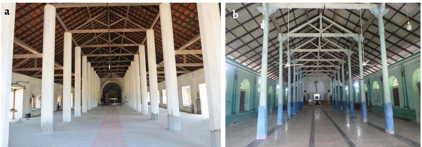
Figure 10. Restoration works in: a) Our Lady of Assumption Church in Parappankandal, Mannar, with new concrete columns; b) St Anne's Church in Keerimalai, Jaffna, with an asbestos sheet roof covering, cement plaster on the walls and new mosaic floor (photos: Joaquim Rodrigues dos Santos).
