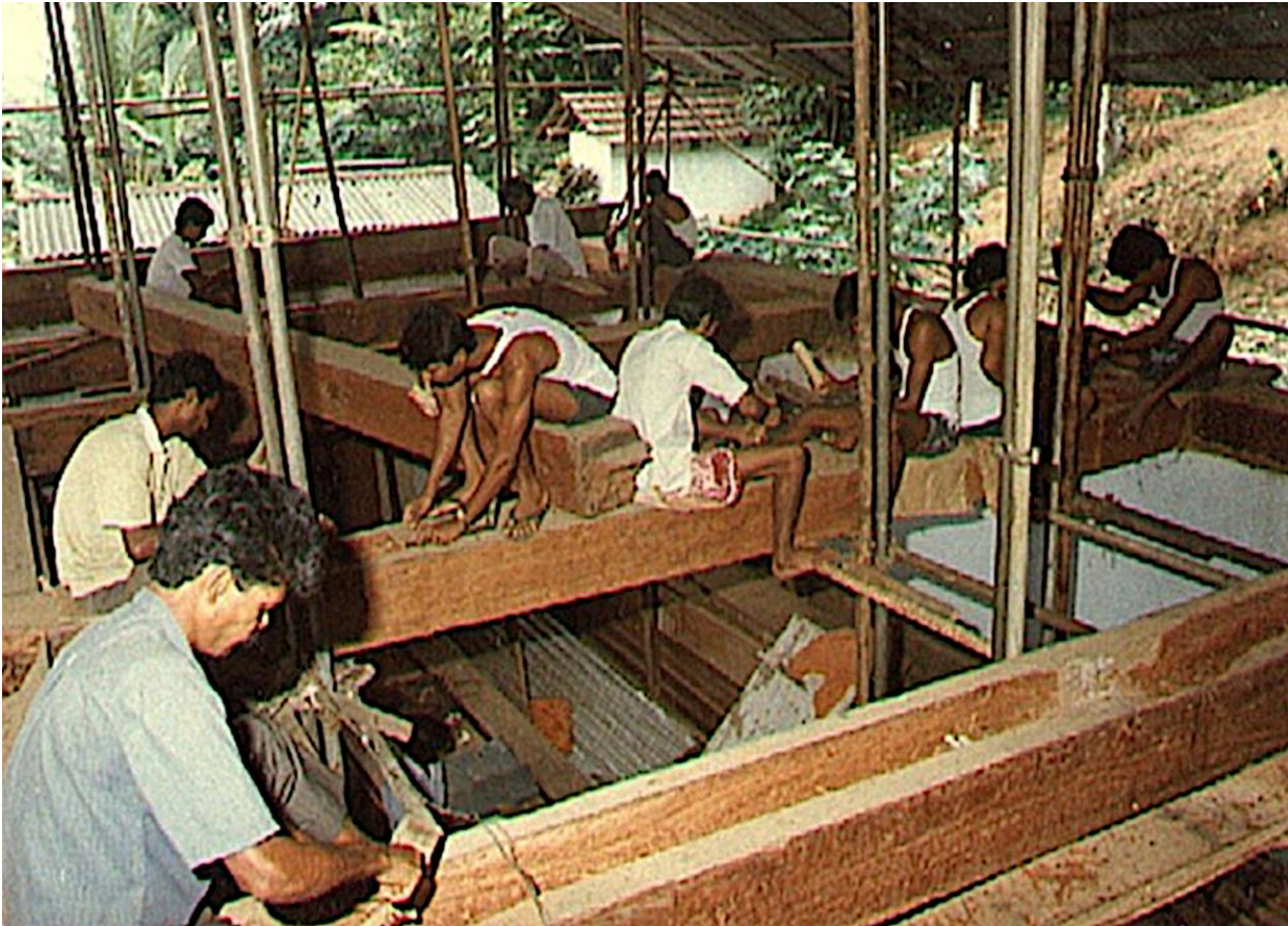
Figure 11. Restoration works on a historic monastic building, famous for its wooden architecture, in the 'Mahavihara' Buddhist Monastery in Kandy (photo: Jayatissa Herath).
