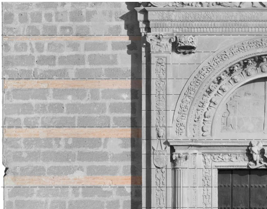
Figure 10. Detail of the main portal: continuity of stone bed joints thanks to the rows of brick.
