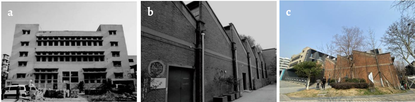
Figure 9. Nanjing Yarn-dyed Fabric Mill: a) from the perspective of Jianzi Alley; b) view of the industrial buildings with the zigzag roof; c) Jinling Art Museum.
