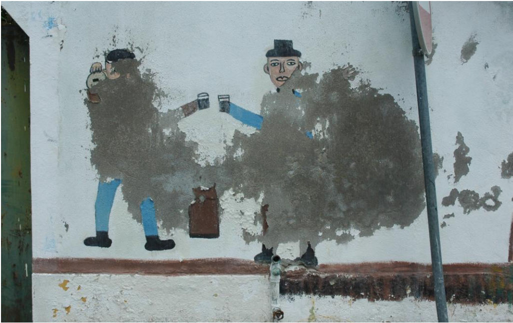
Figure 3. Mural painted in 2012, in extremely deteriorated condition and at risk of total loss, due to the detachment of the paint layer.
