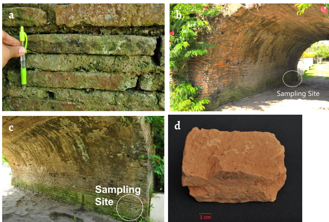
Figure 3. Archway ruin: a ) Portion of the brick masonry wall where the sample fragment was retrieved; b ) View of the front portion of the inner archway facing the east side; c ) View of the back portion of the archway facing the west side (the approximate sampling site is indicated); d ) The brick fragment, where the representative sample was obtained and tested with the different analytical techniques (photographs: J. C. Cayme, April 2014).
