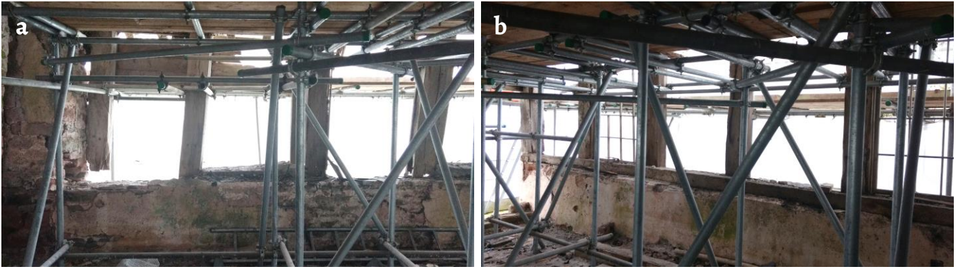
Figure 7. Drying loft: a) East wall; b) West wall (2017).
