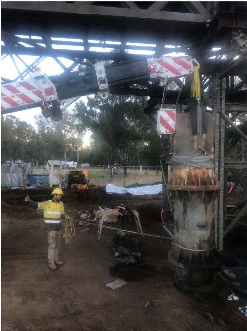
Figure 7. Pier removal using mobile crane (photo: A. Rosnell, 2021).
