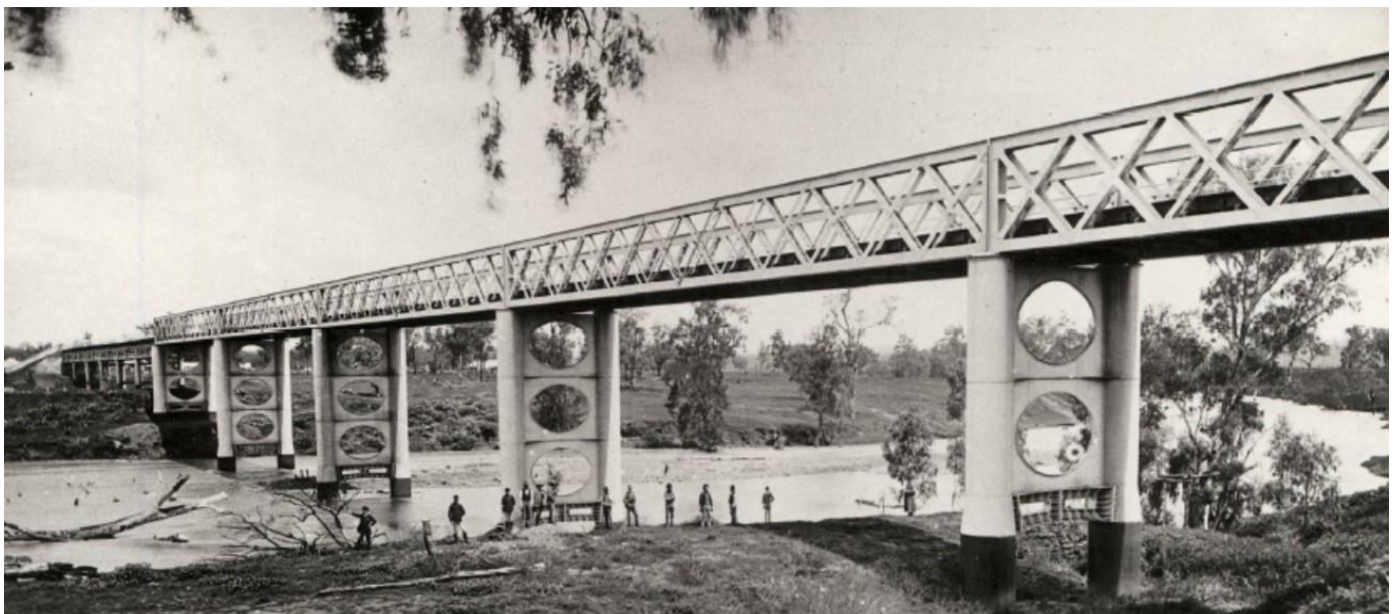
Figure 1. The bridge at time of opening. Note that the approach spans are to the left side of this image after the main truss spans (Photo: NSW Department of Public Works).
