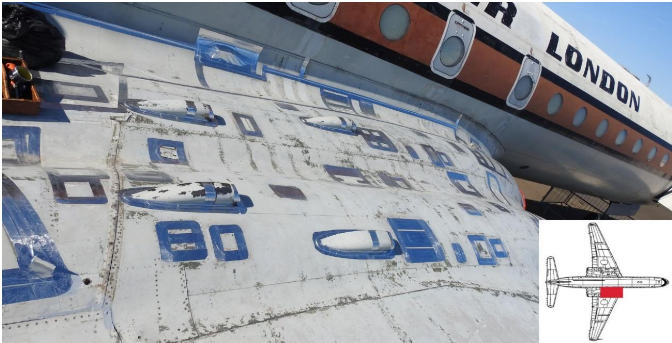
Figure 6. New bitumen based flashing and aluminium foil adhesive tape covering openings and gaps on top of the right wing.
