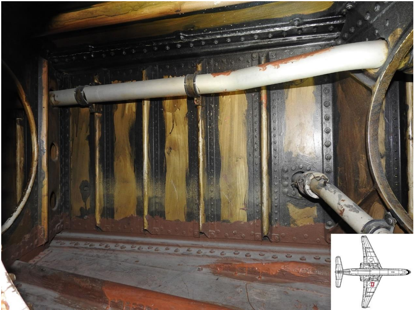
Figure 7. View of the right front main spar.
