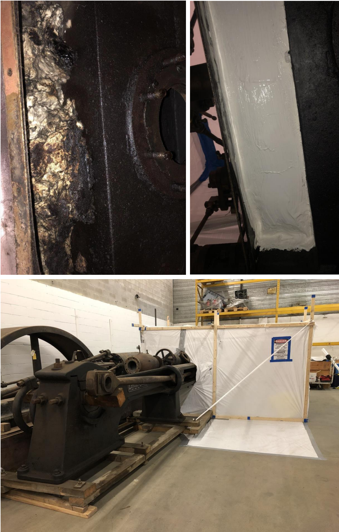
Figure 2. Treatment of asbestos in the Corliss steam engine (Artefact number 1980.0526) by specialised contractors: a) detailed view before treatment; b) detailed view after treatment; c) during treatment showing the custom-built enclosure.
