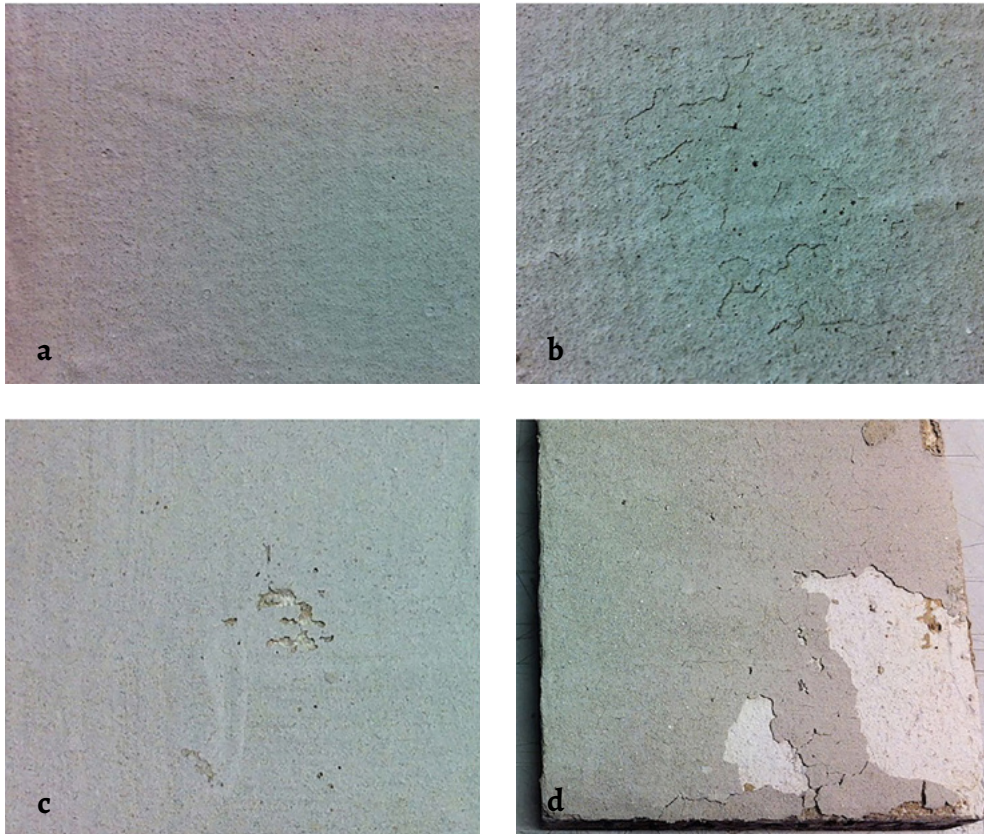
Figure 9. Observed behaviors on the test samples after the water abrasion test: a ) no apparent effect (test sample IB); b ) erosion (test sample I); c ) perforation (test sample IA), d ) loss (test sample I+A).
